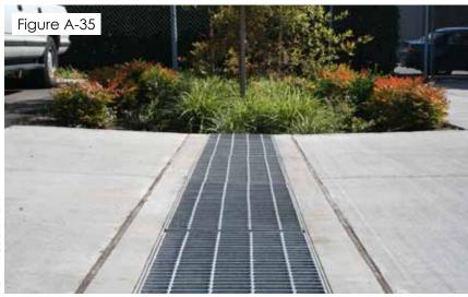
A heavy duty steel trench drain channel conveys surface runoff to a landscaped swale.
