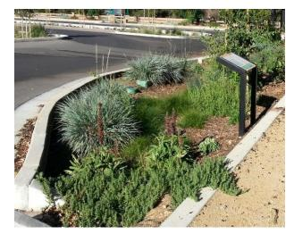
Figure 1. The City of Atascadero Zoo LID Parking Lot Project includes vegetated bioretention facilities that capture, treat and infiltrate stormwater runoff. Signage and pathways promote an educational experience.
