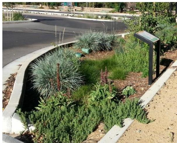
Figure 1. The City of Atascadero Zoo LID Parking Lot Project includes vegetated bioretention facilities that capture, treat and infiltrate stormwater runoff. Signage and pathways promote an educational experience.
