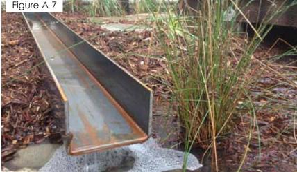
This metal runnell allows water from a building downspout to be
