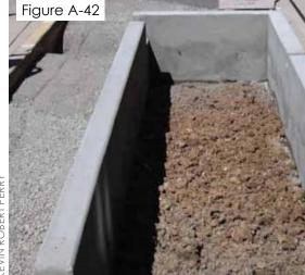
The native soil condition in this planter is scarified to break up any compaction from the excavation process.
