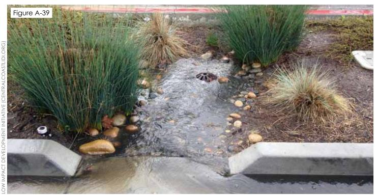
This overflow inlet is incorrectly placed flush with the soil surface and in line of the water flow path. No water can interact with the landscape.
