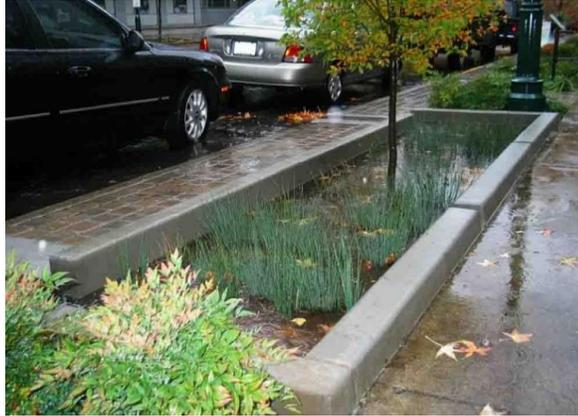
Figure 8. Space constraints may call for a more compact design such as a bioretention planter. For the same performance objective, simple rain garden type designs tend to cost less than the more engineered bioretention or biofiltration type designs. However, this will depend on several factors including cost of land, materials used for the project and long-term maintenance requirements.
