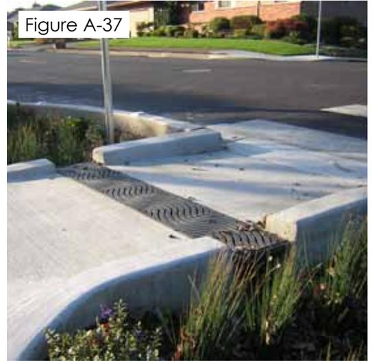
A trench drain connects two stormwater planters through a sidewalk zone.
