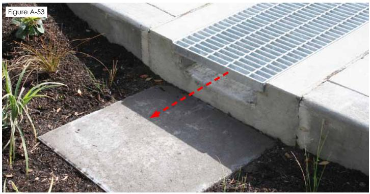
This concrete splash pad dissipates energy from as water drops vertically from the trench drain.
