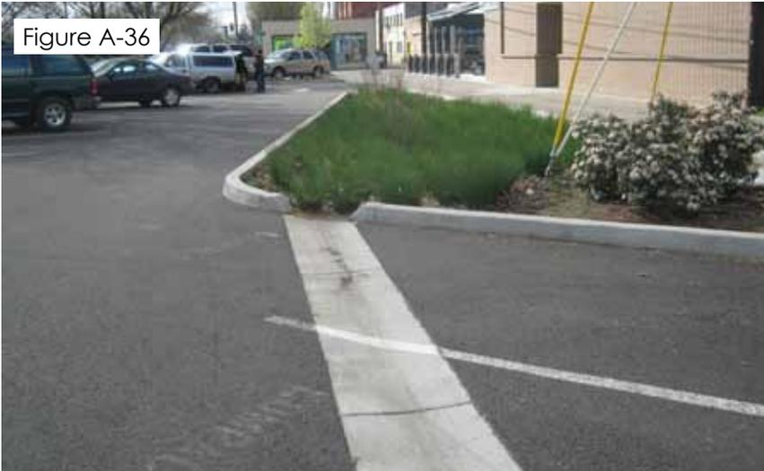
A shallow concrete valley gutter conveys surface runoff from a parking lot into a rain garden.
