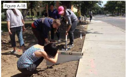
Students helping to build a swale are using a wood template that determines an exact 4:1 soft grade transition from the sidewalk.
