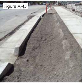
The final grade of the soil is lightly compacted by a roller or feet only.
