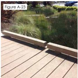
Where there is more that 6" drop in grade, low-profile edge rails can be used to protect pedestrians.
