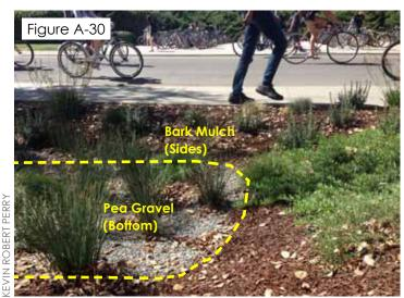
Using pea gravel at the bottom of stormwater facilities can act as a mulch as well as for energy dissipation. Bark mulch can be used along side slope conditions.
