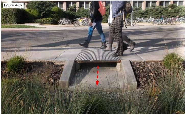
This concrete forebay at the end of a trench drain helps slow runoff and collect sediment before it enters the landscape.
