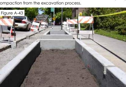
New imported topsoil is placed and mix with the native soil condition.
