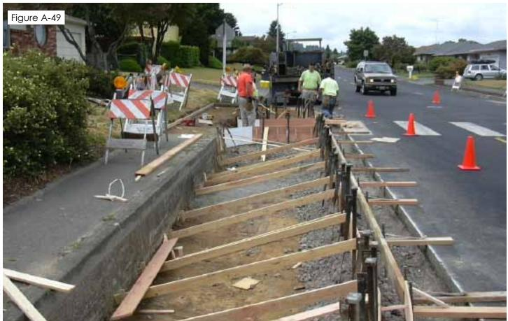
Installation of a deep curb to prevent lateral migration of stormwater into the street subgrade.
