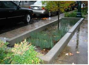
Figure 8. Space constraints may call for a more compact design such as a bioretention planter. For the same performance objective, simple rain garden type designs tend to cost less than the more engineered bioretention or biofiltration type designs. However, this will depend on several factors including cost of land, materials used for the project and long-term maintenance requirements.
