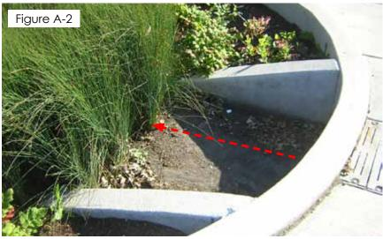
edges. Note that the layer of pea gravel to dissipate energy.
