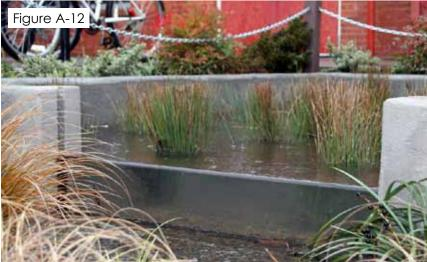
A clear plexiglass check dam is placed within a rain garden to retain exactly a maximum of 6" of runoff.
