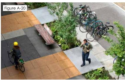
Metal grates are used as pedestrian bridges to cross a school's stormwater planter.
