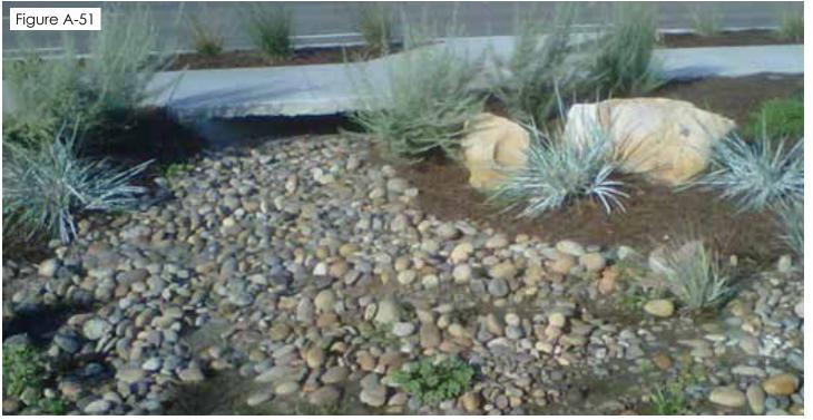
Example of excessive use of decorative cobble which fills with sediment, reduces infiltration, and is challenging to maintain.
