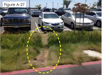
With poor circulation design, people have trampled this vegetated swale to the point where the landscape is beginning to die and soil is being compacted.
