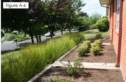
These school building downspouts convey runoff with a concrete runnel away from the building to a stormwater planter.
