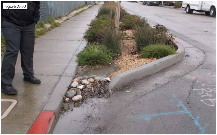
Intended to dissipate the energy of flowing water, this incorrect placement of river rock cobble at the entry curb cut is creating a sediment dam and is actually blocking runoff from entering the landscape.
