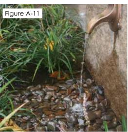
A downspout scupper within a building column allows runoff to enter a rain garden.
