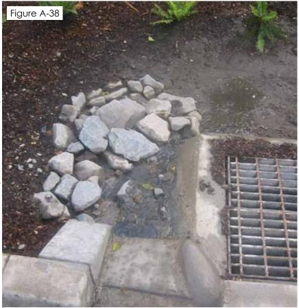
This overflow inlet incorrectly placed against a curb cut forcing water to enter the overflow before it enters the landscape.
