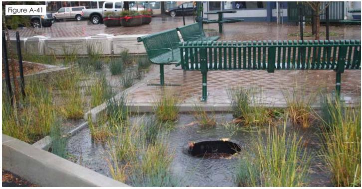
A rain garden with a series of weirs that allow for the brief ponding of water during storm events.
