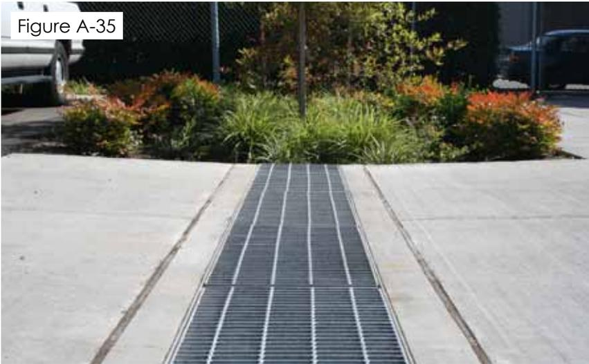
A heavy duty steel trench drain channel conveys surface runoff to a landscaped swale.
