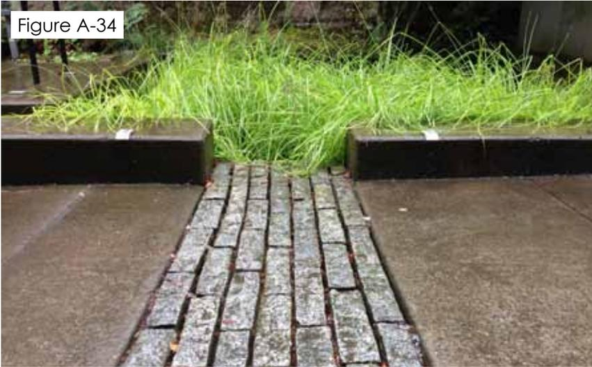
The gaps between granite pavers conveys surface runoff into a stormwater planter.
