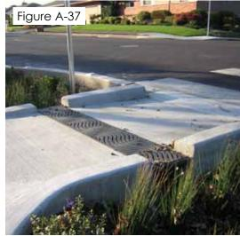
A trench drain connects two stormwater planters through a sidewalk zone.
