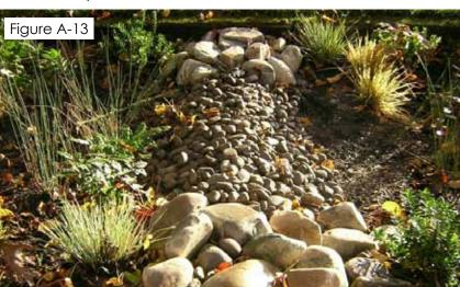
Simple check dams made of different sizes of stacked rock can help slow the flow and retain water upstream.
