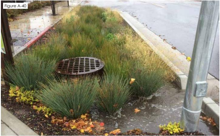
A bioretention system with correct curb cut placement and raised overflow inlet elevations to allow the brief ponding of water.
