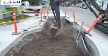
Bioretention construction showing the placement of soil. Note that heavy equipment is located outside the facility to avoid any soil compaction. Also note the vertical liner installed to prevent lateral stormwater movement toward the adjacent street.
