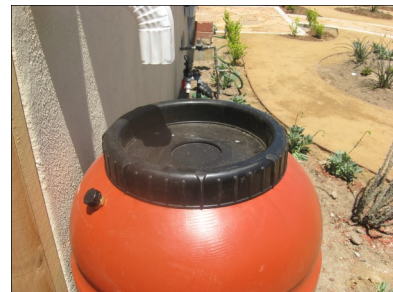
Rain barrel overflow spigot.
