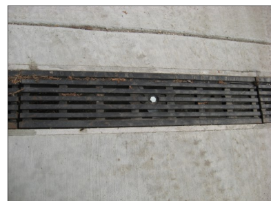
Trench drain at base of driveway.
