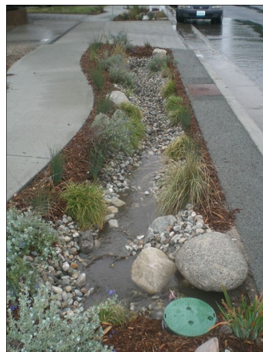
Parkway swale with stormwater.
