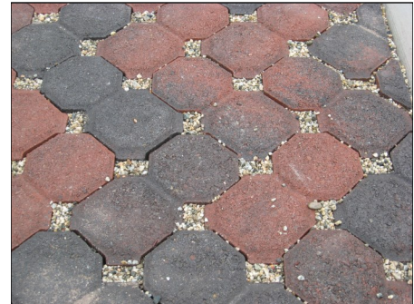
Permeable pavers in driveway.
