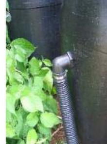
**During heavy downpours, rain barrels fill faster than a garden hose overflow can output excess water. Water can overflow through the top and puddle by your foundation. Over time this can damage substructures.**
